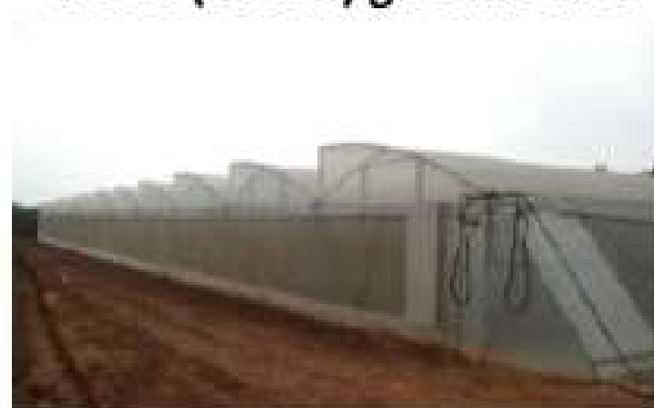
Multi bay (span) greenhouse
