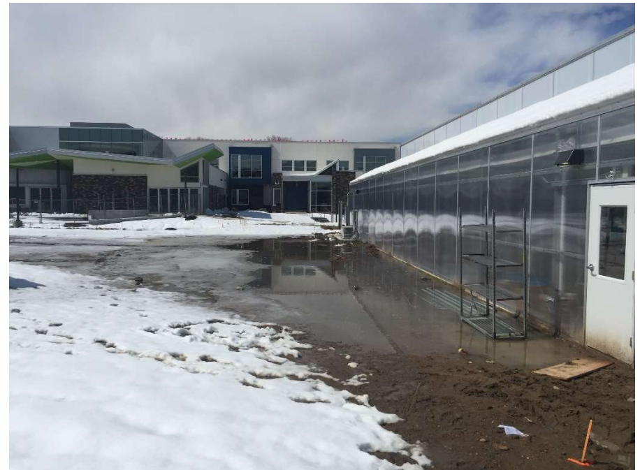
Water pooling outside greenhouse can seep in and also be a vector for pests
