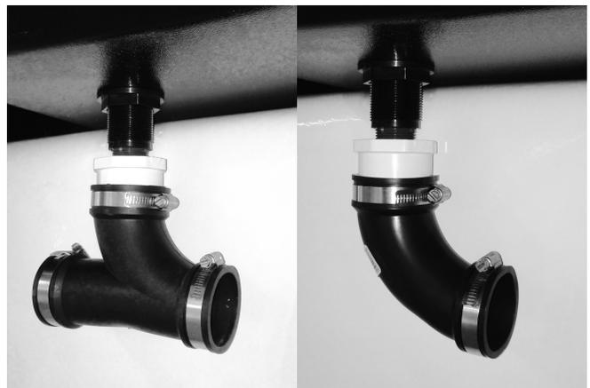
**18B: Insert Fernco 90 black rubber drain pipe onto bushing on last bed in run (furthest from fish tank)**
