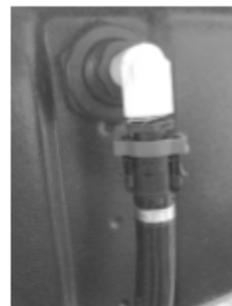
Distribution Backbone attached to Quick Loc socket
