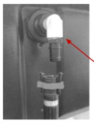
Assembled Threaded elbow with Quick Loc connector
