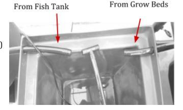
12D: Push DB sections from fish tank and grow beds together on the "T" coming from the DB section in the fish tank
