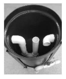
Step 9F: Insert ½" pipe through holes in Stilling Well and position in SFF over the outflow standpipe Parts Needed:
